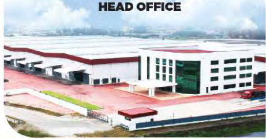
ASTINO METAL PENANG HEAD OFFICE
