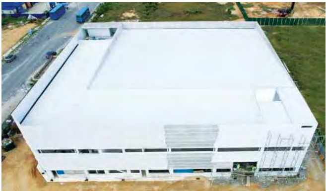
Aluzinc AZ150 0.47mm TCT High Rib PU Foam 25mm
