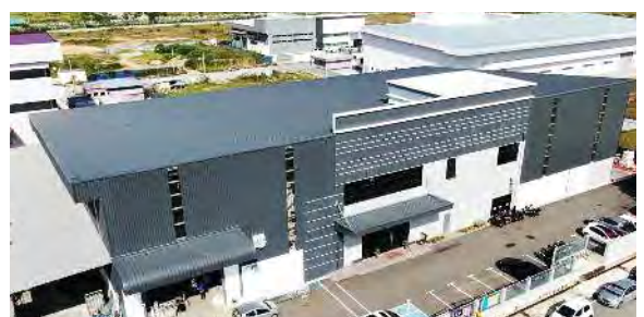
CG SOLUTIONS ENTERPRISE SDN. BHD. Realcolor Primero 0.40mm TCT Superior Rib PU Metal 20mm in Volcanic Grey
