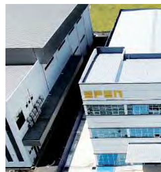
SPEN INDUSTRIES SDN. BHD. Aluzinc AZ150 0.35mm TCT Superior Rib PU Aluminium 25mm
